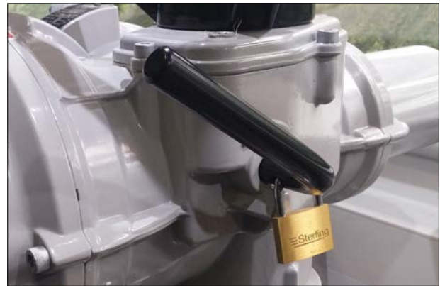
Fig 7.1. IQ3 hand-auto lever padlocked
