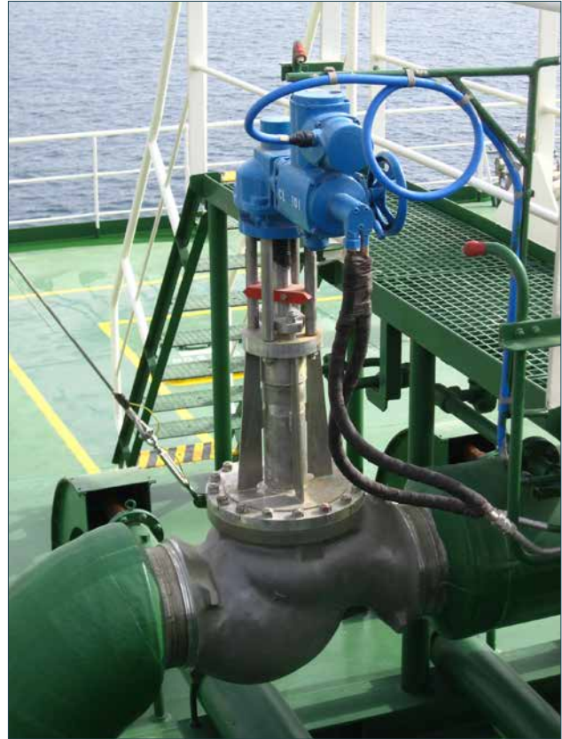
4H1.100 multi-turn hydraulic actuator, 1000 Nm rated torque, mounted on a DN300 cryogenic globe valve on one of the LNG vessels where the actuators are now operating.
