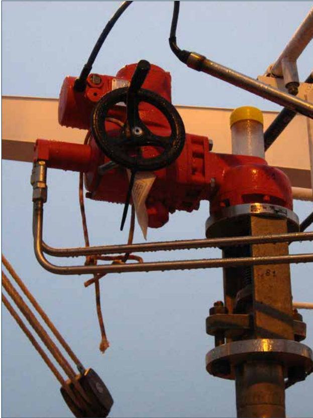
4H1.050 multi-turn hydraulic actuator, 500 Nm rated torque, mounted on a 12" - Class 150 globe valve on an LNG vessel.
