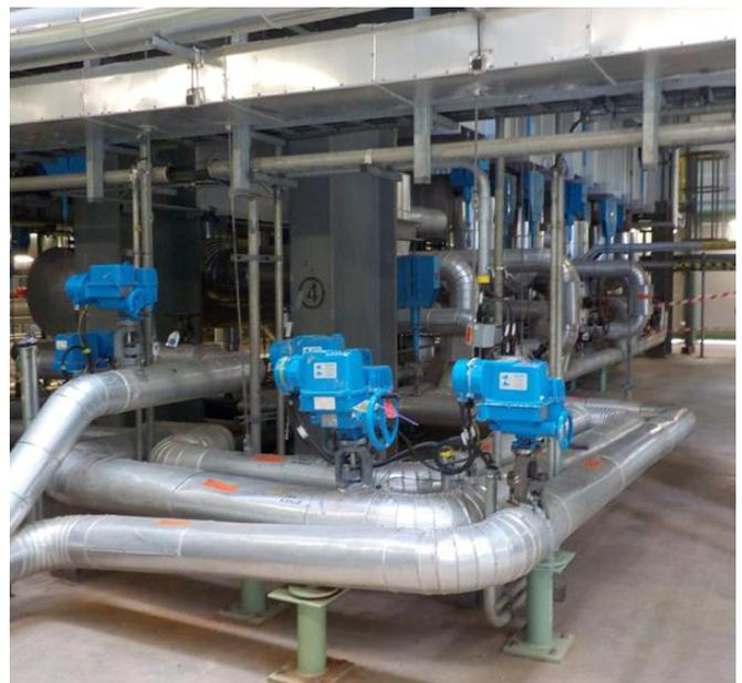
*Fig 1 – An area of blowdown valves prior to the upgrade.*
