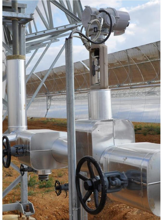
*A control valve on heat transfer fluid pipework retrofitted with a Rotork IQTF linear actuator to provide precise remote control of the HTF temperature*
