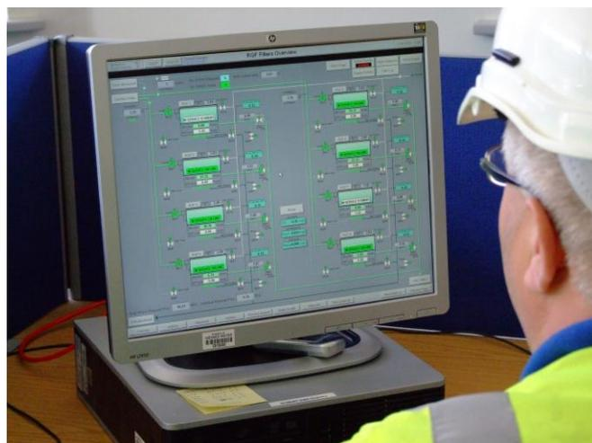
*SCADA screen at Maundown, monitoring the operation of rapid gravity filters*
