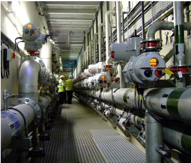
*IQT actuators controlling the backwashing sequences on the membrane plants at Swanage*
