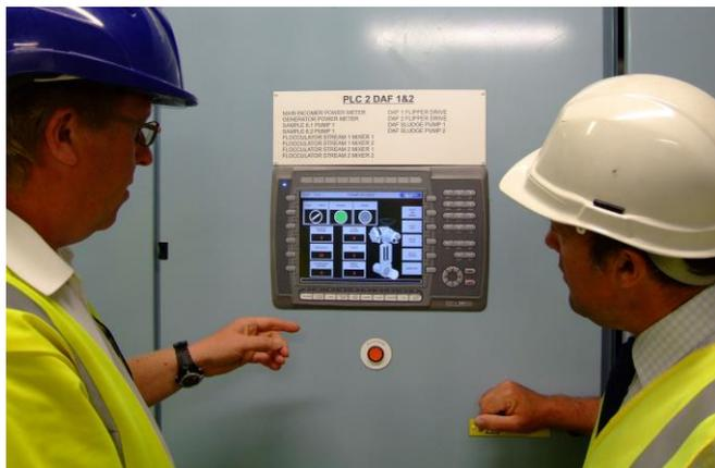
*HMI screen at Maundown. The Rotork actuators can be interrogated, monitored and controlled at these stations*
