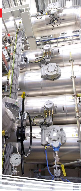
Safety is of primary importance and for this reason virtually all the ball valve installations are of double block and bleed design, the largest weighing in at eight tonnes. Security against leakage is vital for the accuracy of the metrology as well as safety.
