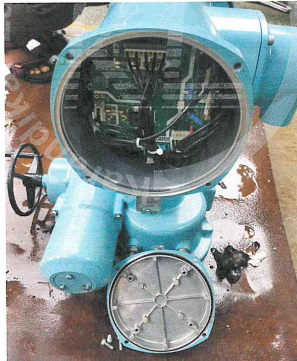
Pictute2: No ingress of powder & water observed
