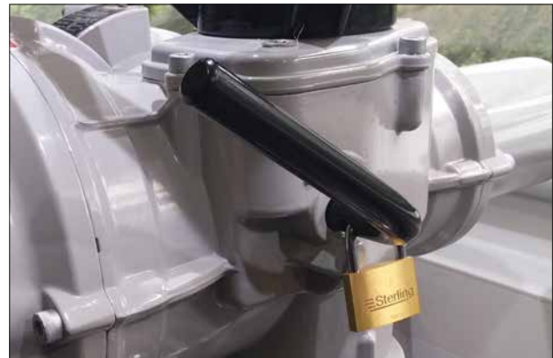
Fig 7.1. IQ3 hand-auto lever padlocked
