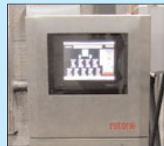
The Rotork-designed cabinet houses the Pakscan master station and displays the information provided by InVision software.
