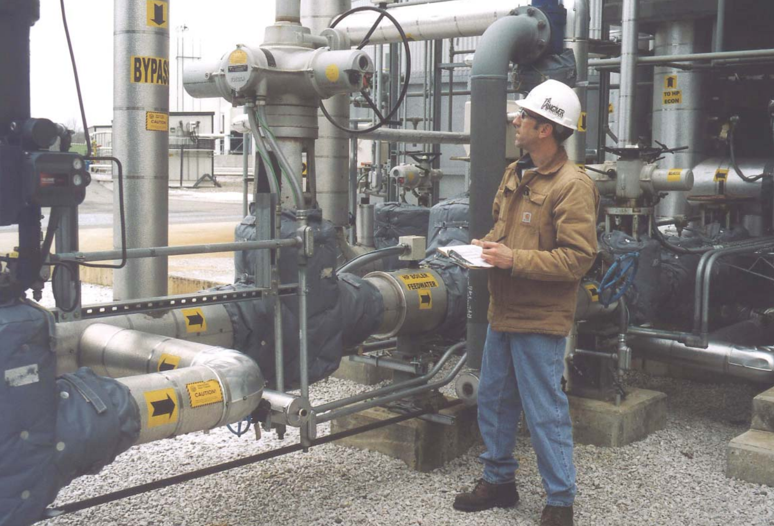
Rotork IQ actuators installed at a power station in the USA.
