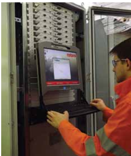
Fig 5 Cabinet-mounted Rotork SVM units. The integrated computer enables the operator to analyse partial stroke testing data and diagnose potential issues.
