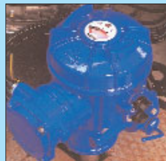
One of the Rotork AQ 115 actuators installed at Tottiford Reservoir.
