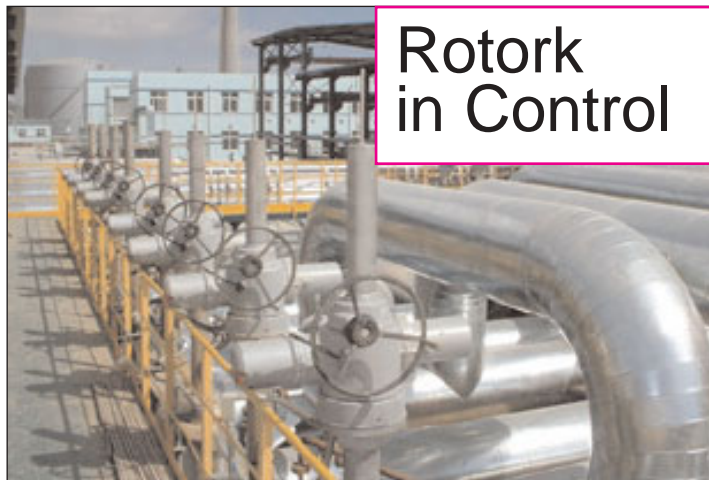
Rotork IQ90 valve actuators installed on the Da Xie Tank Farm manifolds.
