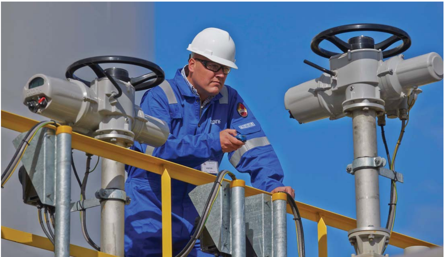
Fig 3 – The diagnostic information available from the IQ datalogger can be extracted from the actuator using the secure Bluetooth® hand-held Setting Tool Pro.
