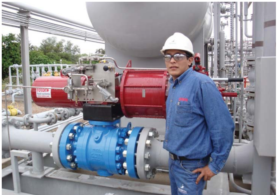
Fig 4: Three progressive levels of cover meet differing demands and are designed to seamlessly integrate with existing maintenance procedures and strategies.
