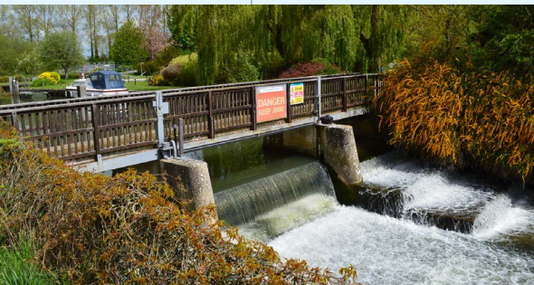
Buscot Weir prior to the upgrade.
