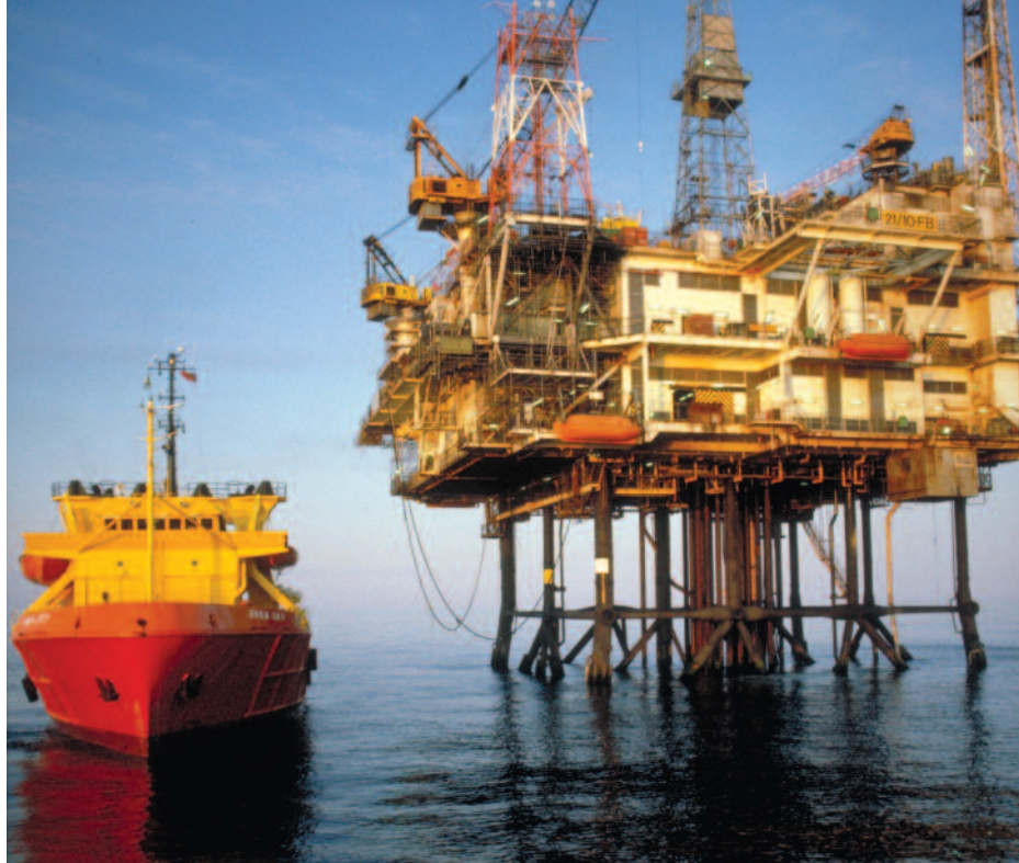
Safety Integrity Levels are targets applied to the reliability and performance of the safety systems used to protect hazardous activities such as hydrocarbon refining or production.
