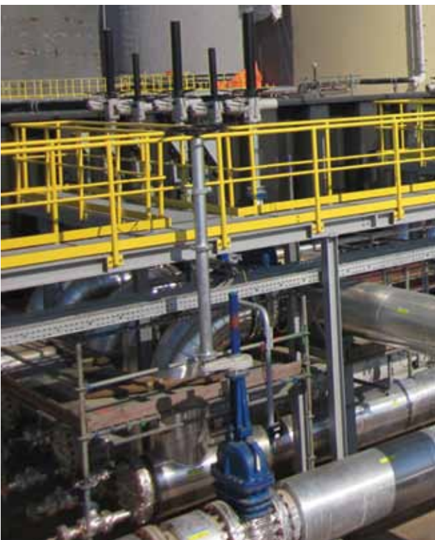
Fig 3: IS range spur gearbox/stem extension installation.
