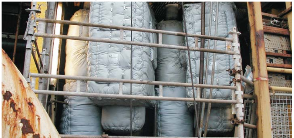
A semi-rigid fireproofing installation.
