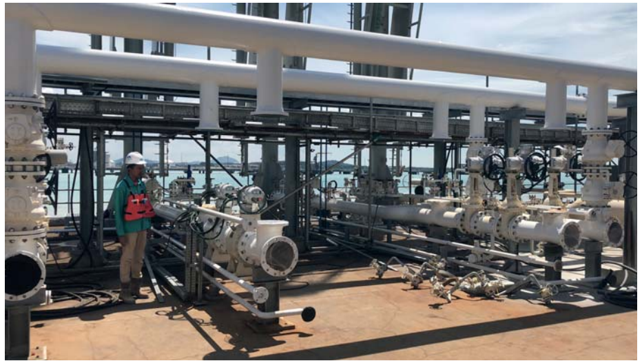
Some of the IQ3 actuators at the terminal during installation.
