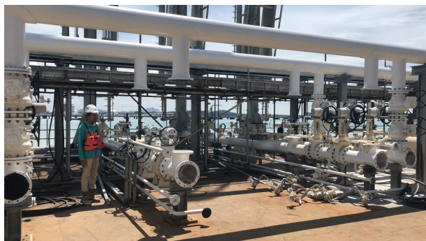
Figure 1. Intelligent actuators in operation at a terminal.
