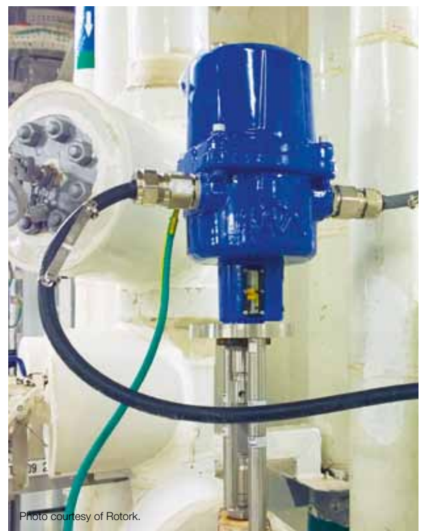
One of the Rotork CMA actuators installed on the CLOV HVAC system.
